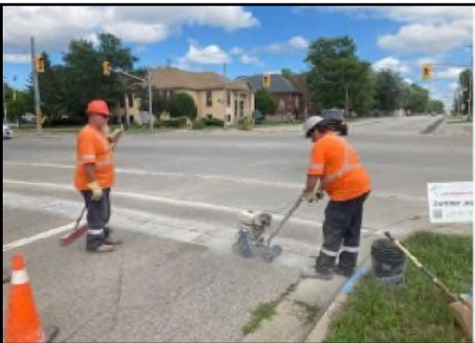
Above: Vic O'Leary(right) and Wayne Bradburn are working at the intersection of Hill and Lyndoch Streets in Corunna. They are preparing the road surface for the reapplication of pavement markings. Works Dept. photo
