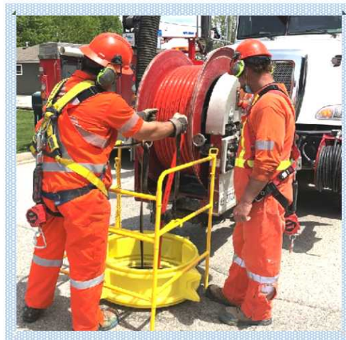
Public Works Water/Wastewater operators Scott Barnes and Aaron Jardine performing sanitary sewer flushing in Port Lambton. Works photo
