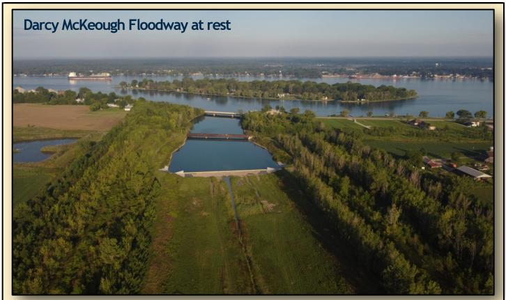
You're looking west along the Darcy McKeough Floodway diversion channel under normal conditions, when its floodgates are open and the channel is above water. It's the largest flood diversion project in Ontario and it limits the flooding risk to Wallaceburg when water levels in the East and North Sydenham Rivers are high.
