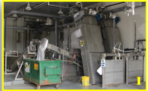
Screen room (inside inlet works building) is where effluent enters the plant.
