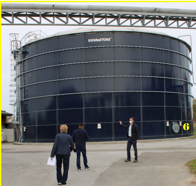
The biosolids storage tank stores the treated sludge until it can be transferred to trucks for disposal via land application during a short period of time each year. The guide for this tour was Brian Black, Director of Public Works.
