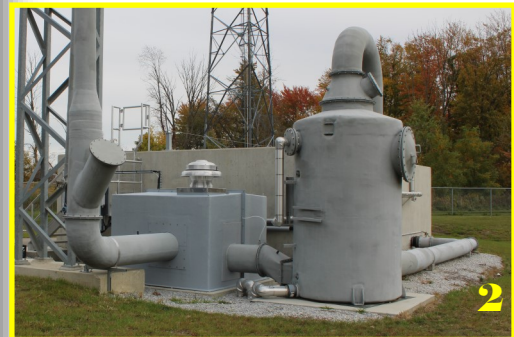
New biofilters treat odorous air from the inlet channel at the front-end of the aeration basins, the aerobic digester, biosolids storage tank vent, and truck loading station.
