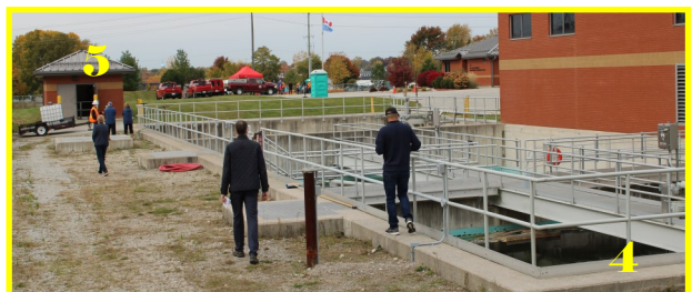
The secondary clarifier tanks, (4) foreground, further treat effluent, which is then separated, and the cleaned water sent to the UV disinfection building (5) for use in the plant. Sludge from these tanks is sent to the biosolids storage tank (6).
