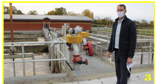
Brian Black describes the function of the aeration basins where effluent is treated by bacteria that feeds on it.
