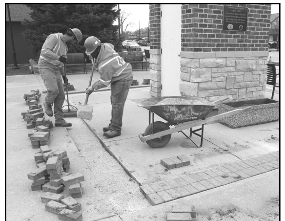
S & S Greenhouse employees Mike Ravenhorst, left, and Damion Gray reset brick paving stones that have heaved and pose a tripping hazard to visitors to the clock tower park. Bonnie Stevenson photo
