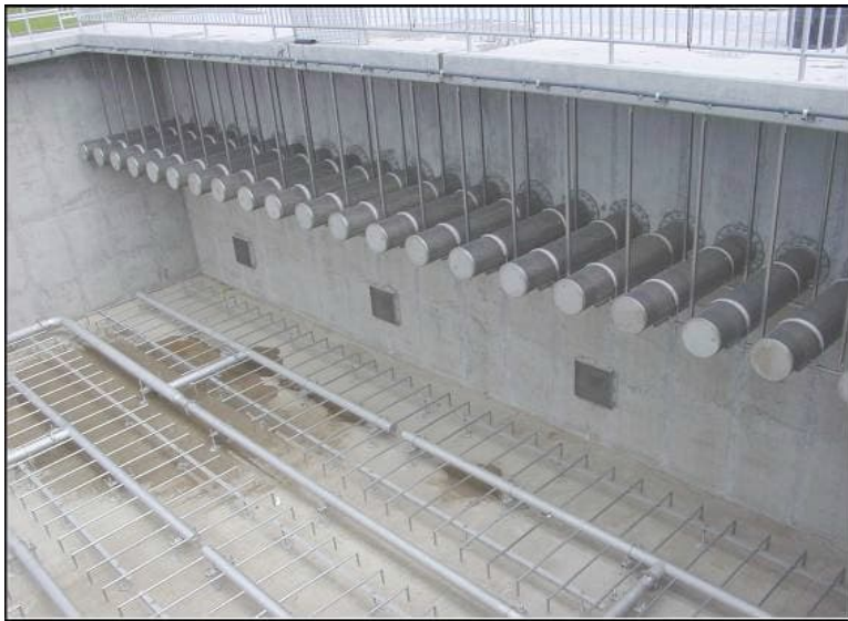
Figure 10-3. Photo of Media Retention Screens
